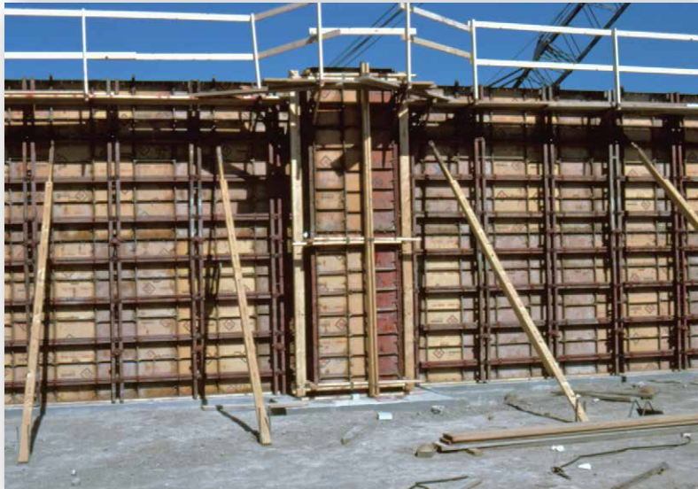
Pilaster Formed with Standard Steel-Ply Components
