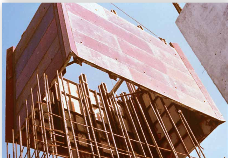
Double Hinged Filler with 90° Inside Corner
