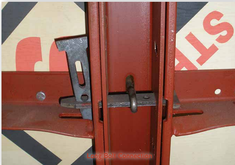
Typical Wedge Bolt Connection
